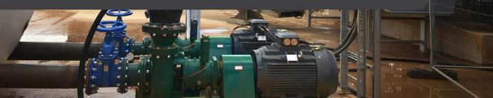
Pioneer standard centrifugal pumps provide superior performance in a variety of high pressure, sewage, trash or dewatering applications. The large stainless-steel impeller eye yields lower NPSHr and improved vapor-handling capabilities, making them ideal for industrial, municipal, agricultural, mining, and oil and gas settings.
